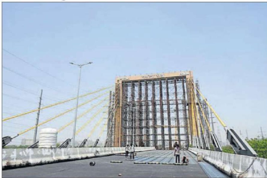
The Parthala flyover in the final stages of work on Monday.
